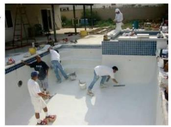
When plastering is completed, the plaster foreman will place a hose in the bottom of the pool and he will tell you what time to turn on the water.
