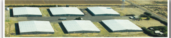
Warehouse Facilities, Eloy AZ. 10 Acres of Buildings, 85 Acres Land
